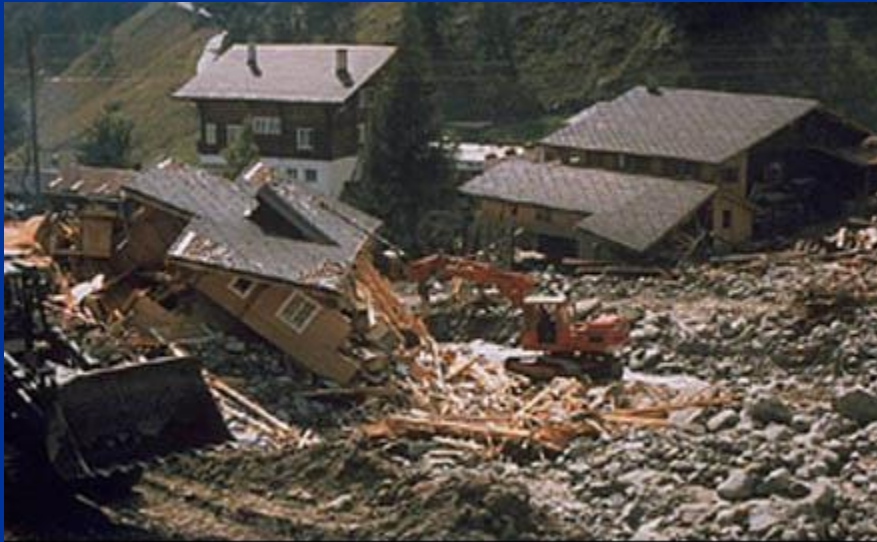
Houses undermined by melting Permafrost
