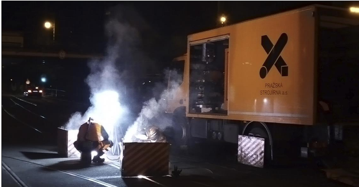
Fig. 7 – Welding and reprofiling of the crossing Výtoň 12.7.2020
