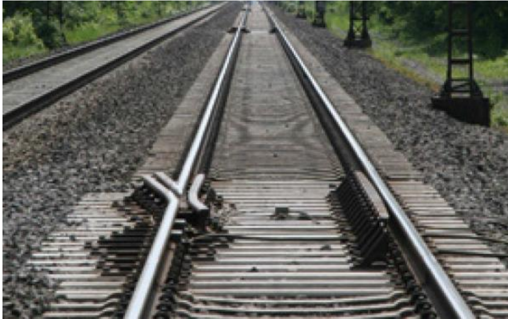
Fig. 2 – Test track for switch frogs near Hannover (picture: [7])
